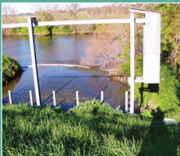
Figure 1 Booms and gates across the river entrance to irrigation farms – a control measure to help protect this farming area from alligator weed
