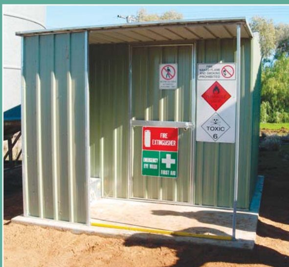
Figure 1 A chemical storage shed that meets Australian Standards, and provides farmers with one centralised, organised and simple management system for pesticides used on farm
