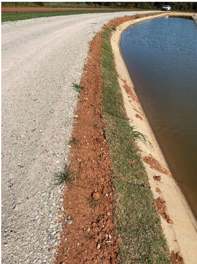
Above: Kikuyu turf 1 month after application
