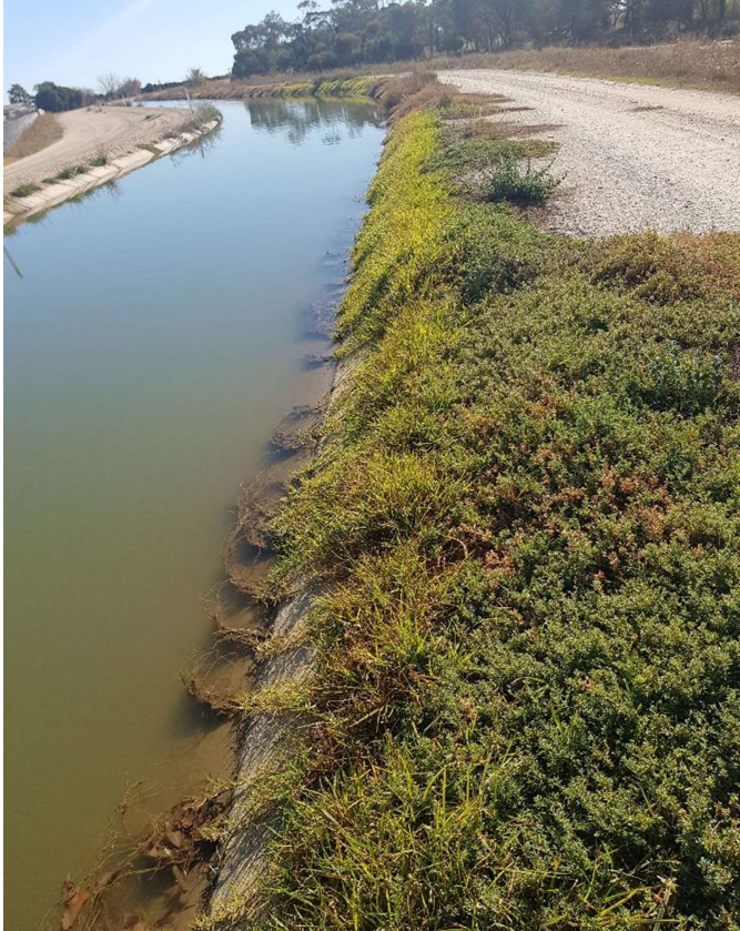
Above: Kikuyu turf at completion of trial
