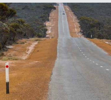
Major roads and highways tend to have wider cleared areas, predominantly for road-user safety. Ravensthorpe, Western Australia. AGRONOMO
