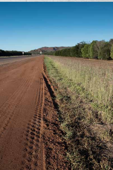
Road verge cleared width tends to increase in less populated areas. East Kimberley, WA. AGRONOMO
