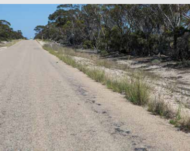
To maintain the integrity of the road base from ingress of water it is important to keep weeds from the edge of the tar. Perennial grasses are a problem because they are hard to control and thrive on the water harvested from the road surface. Grasspatch, WA. AGRONOMO
